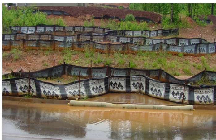
Erosion at construction sites is usually controlled with silt fences.
